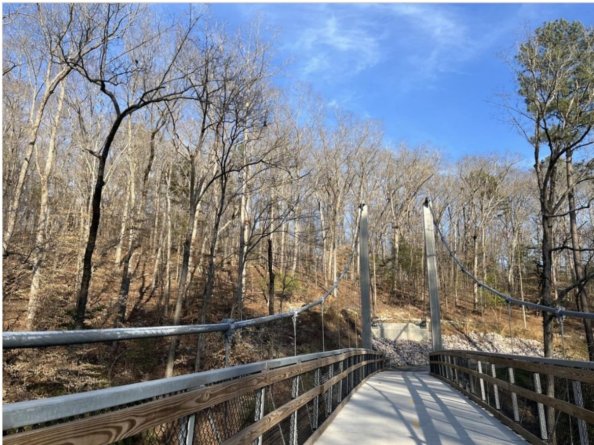
Figure 2. Duraleigh Forest rocky hillside above the suspension bridge on the Crabtree West Greenway, in winter showing the mature deciduous forest at 5000 Duraleigh Road.
